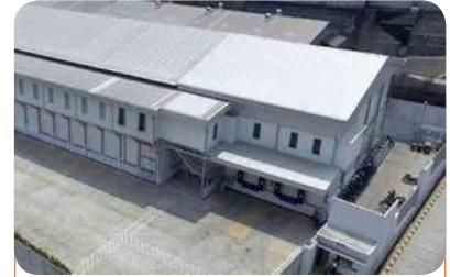
Gudang Logistik Narogong Narogong Logistics Warehouse
