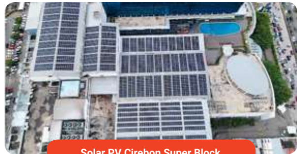
Solar PV Cirebon Super Block
