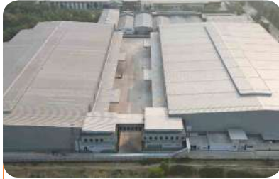
Gudang Logistik Cikarang Cikarang Logistic Warehouse
